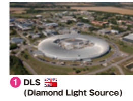
1 DLS (Diamond Light Source) Start of Operations 2007 Circumference 562m Energy 3GeV Beamlines 33
