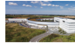
2 SOLEIL Synchrotron Start of Operations 2006 Circumference 354m Energy 2.75GeV Beamlines 29
