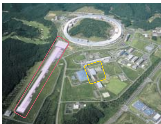
The site where the XFEL facility will be built
